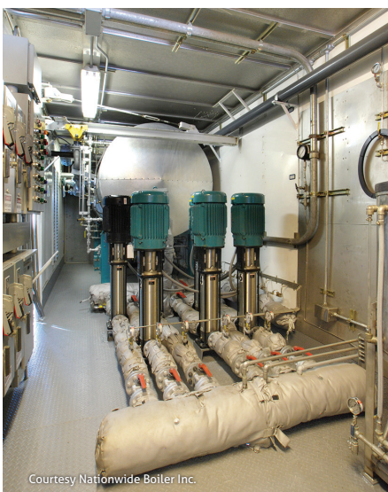
Feedwater pumps inside a mobile feedwater van also equipped with deaerator, water softener, chemical feed system and motor control panel.
