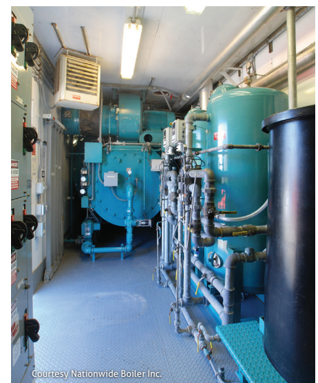
A mobile boiler room typically includes the boiler/burner package, atmospheric feedwater system, water softener, chemical feed system, blowdown separator and motor control panel.
