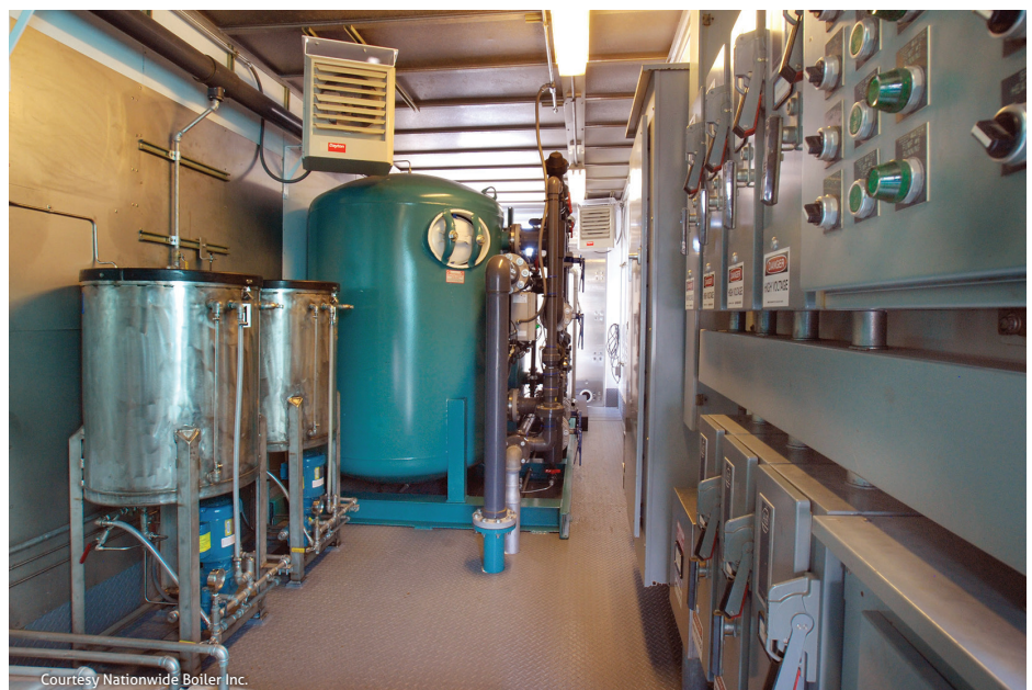
Interior of a mobile feedwater van, the auxiliary equipment often rented with boiler systems.
